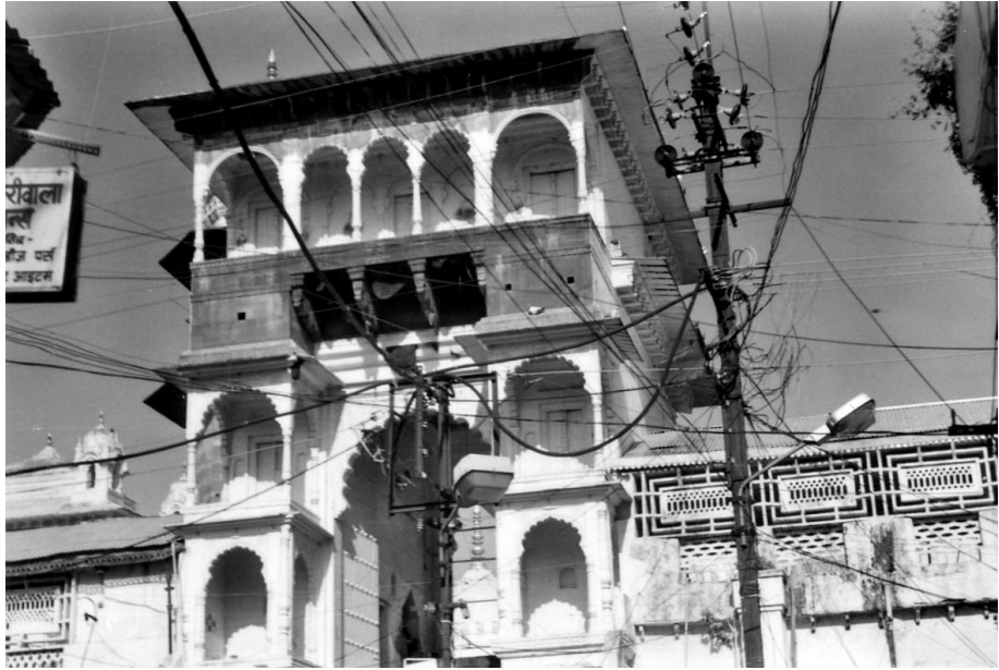
Figure 4: Nawab Qudsiya Begum's Jami Masjid, Bhopal: Entrance Gateway (Image Courtesy: Commissioner, Archaeology, Archives and Museums, Government of Madhya Pradesh, Bhopal)
